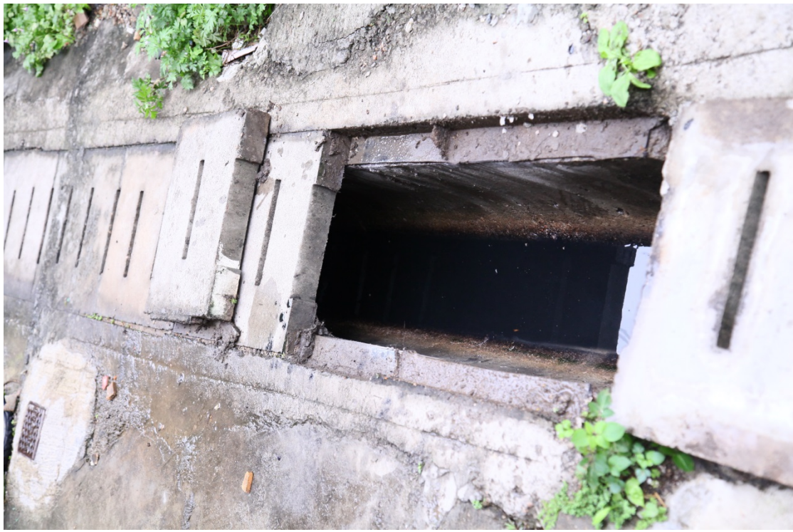
Condition of Drainage
